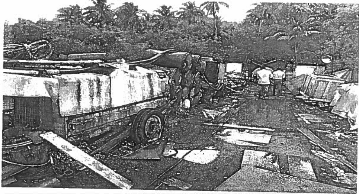
Ship Building Area Belongs to M/s Shaparia Docks and steel Company Ltd
